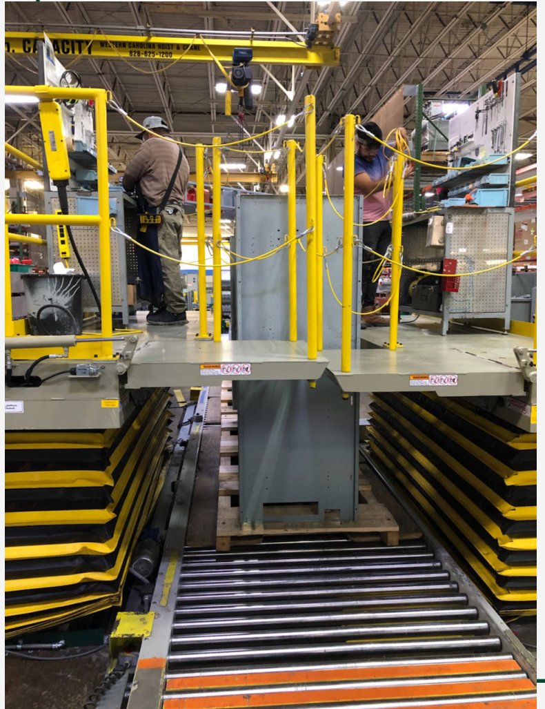
New Assembly using Southworth Lifts
